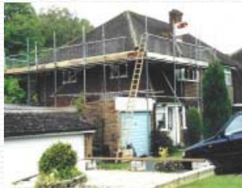
Original view of house before work commenced
