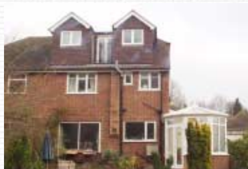
Rear view of bespoke conservatory linked to new dining room behind
